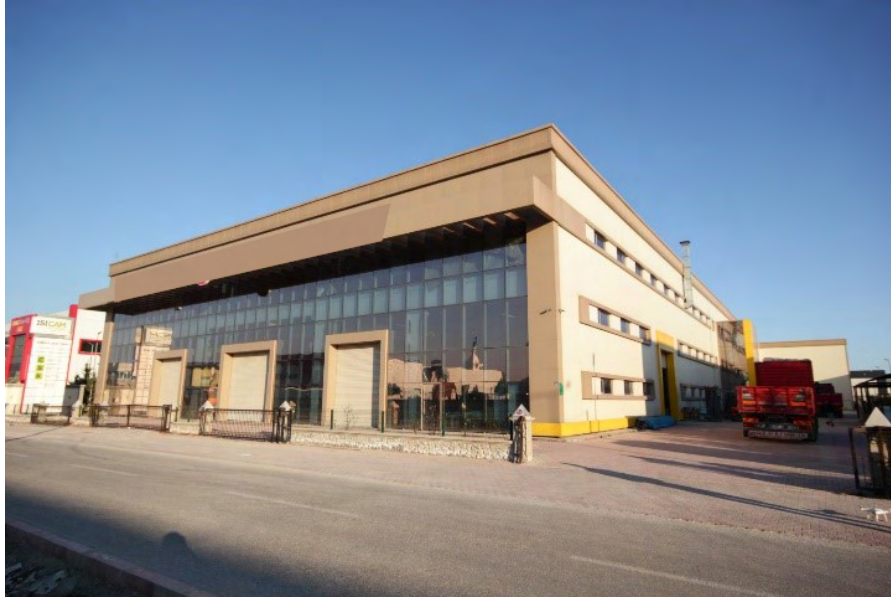
Figure 3: Facade of glass factory.
